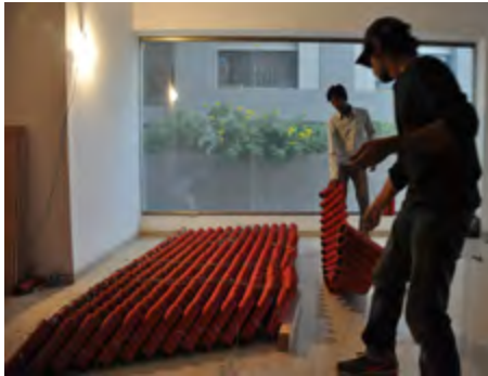
Weaving of a single strip with SS cable.
