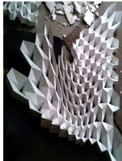
Second layer : A layer of putty applied onto it.
